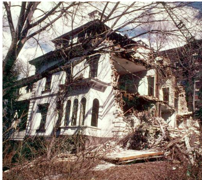
Top: Tiffany-Bowles House; Bottom: demolition, 1980. Courtesy of the Wood Museum of Springfield History
